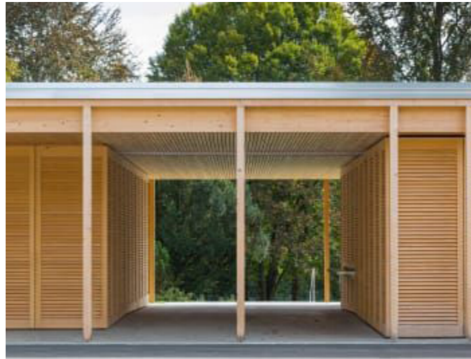
Timber structure forming collonade
