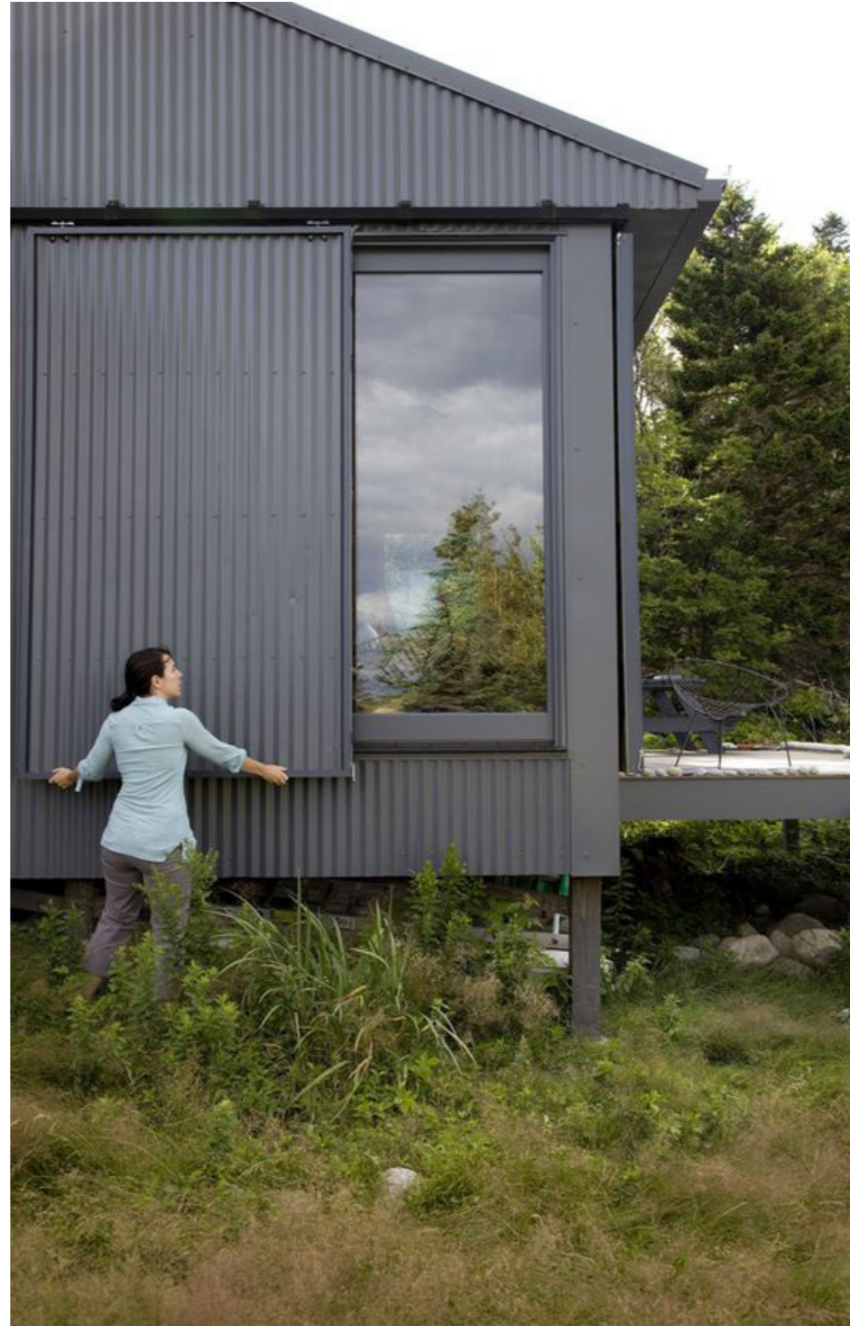
Dark cladding with external door
