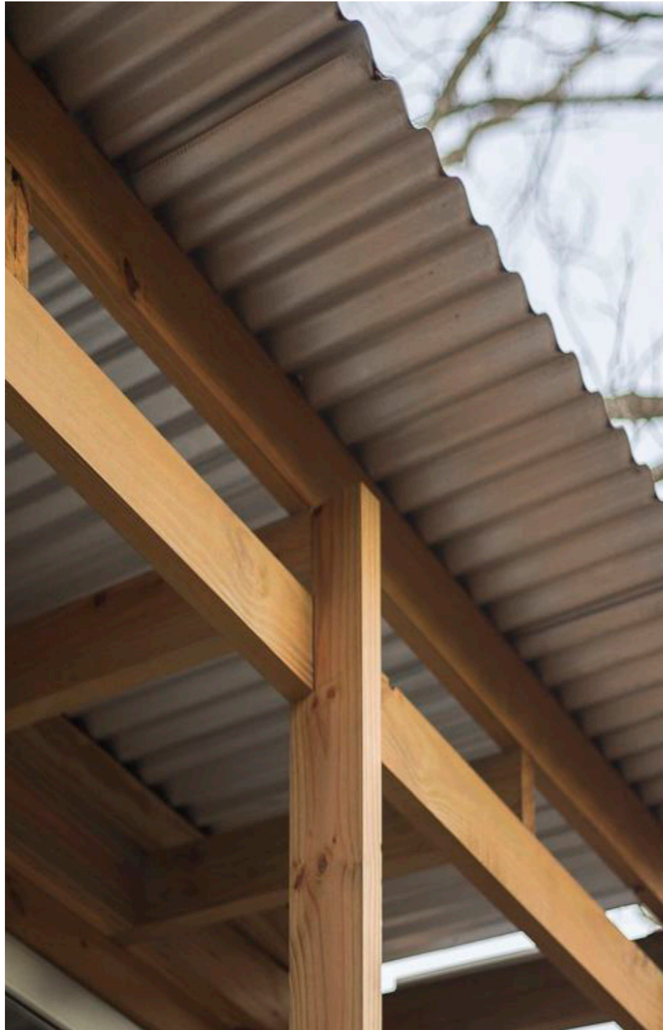
Timber structure and corrugated roof
