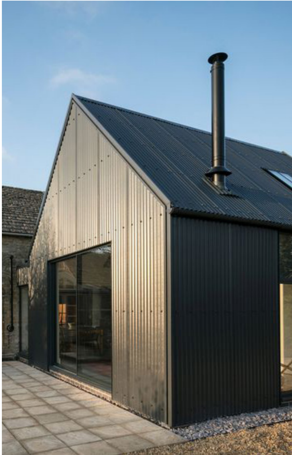
Dark cladding to wall and roof
