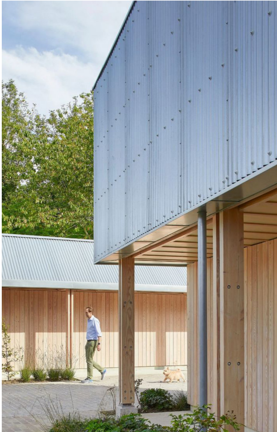
Timber collonade and metal cladding above
