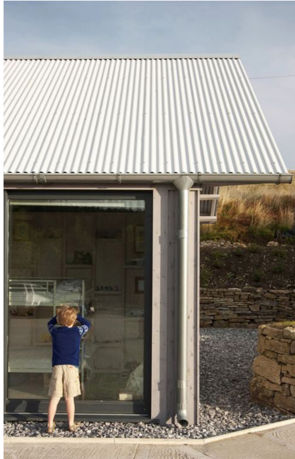
Galvanised corrugated roof with timber cladding below
