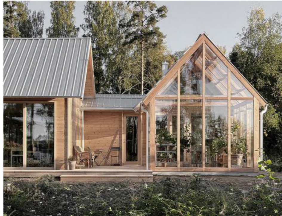
Feature openings and integrated joinery
