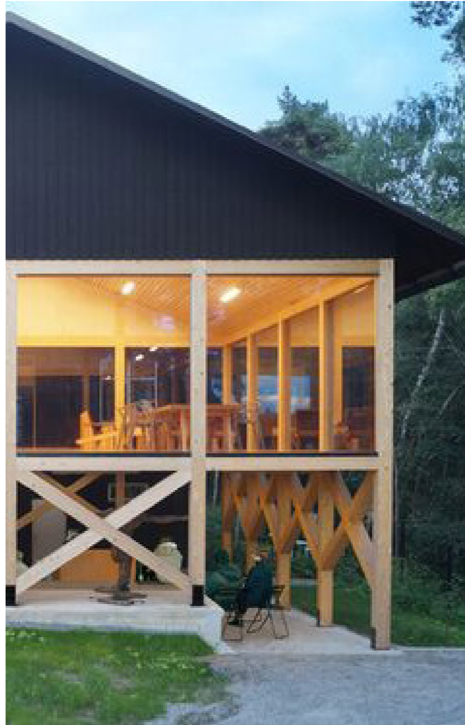
Dark cladding and light timber structure
