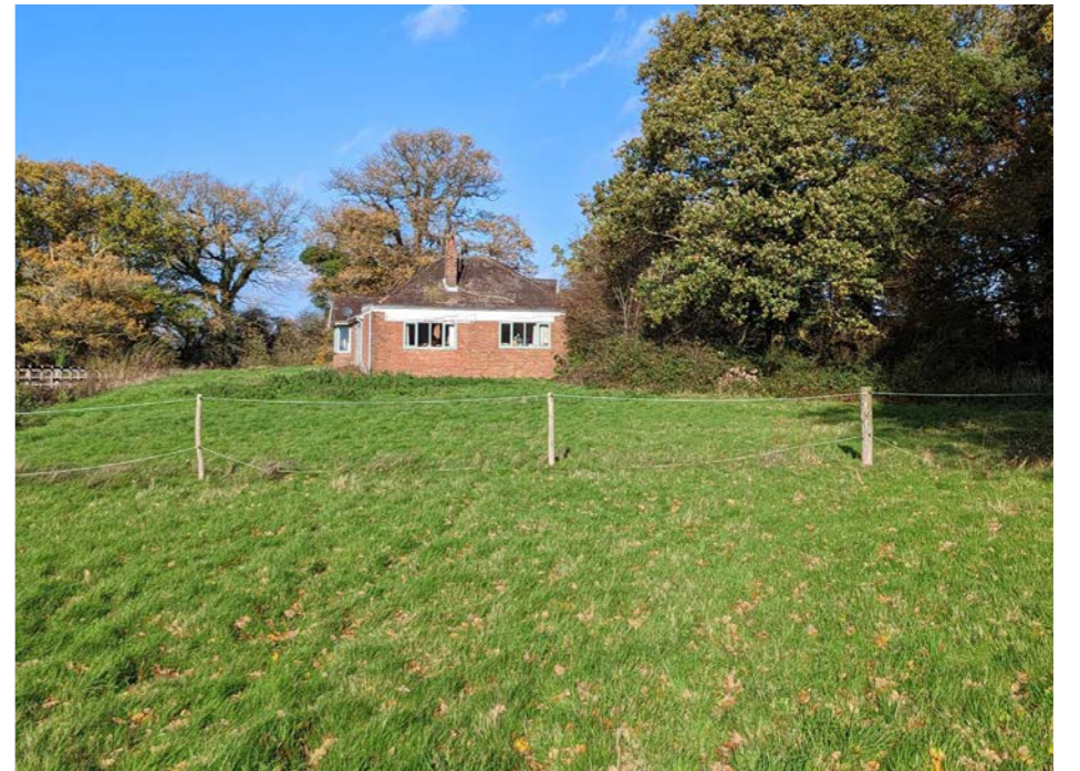
South side of bungalow
