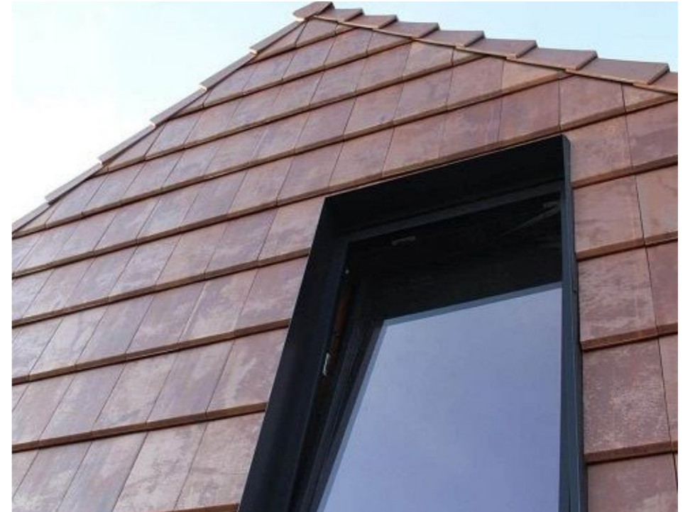
Contemporary window detail in hung tile facade
