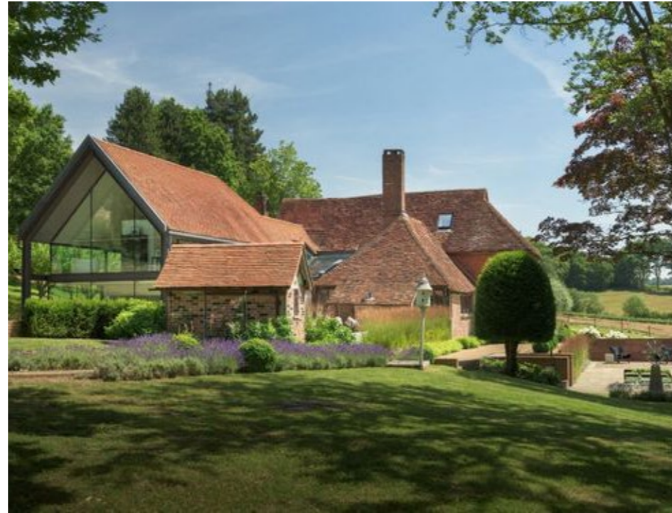
Clay roofs with a modern extension to historic building that's typical to the High Weald AONB
