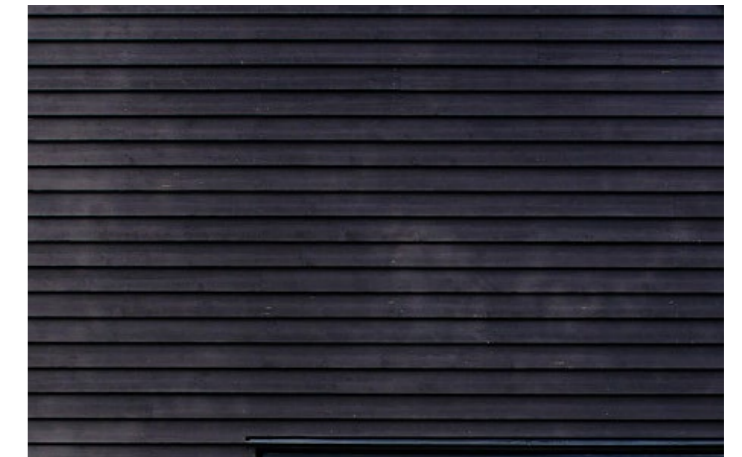
Horizontal timber cladding
