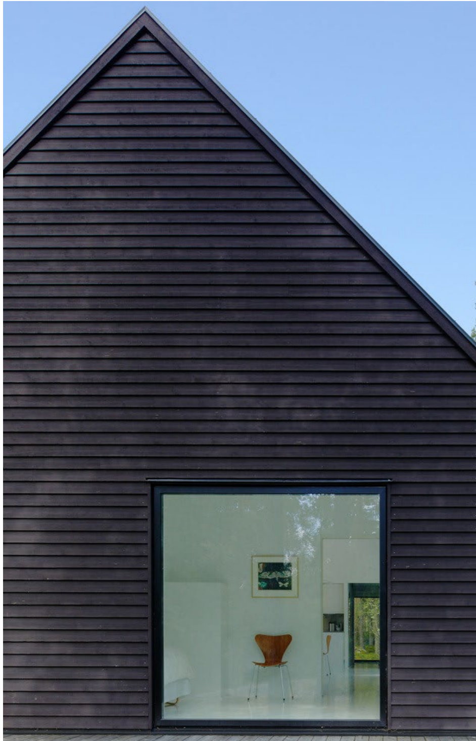
Simple horizontal timber detailing
