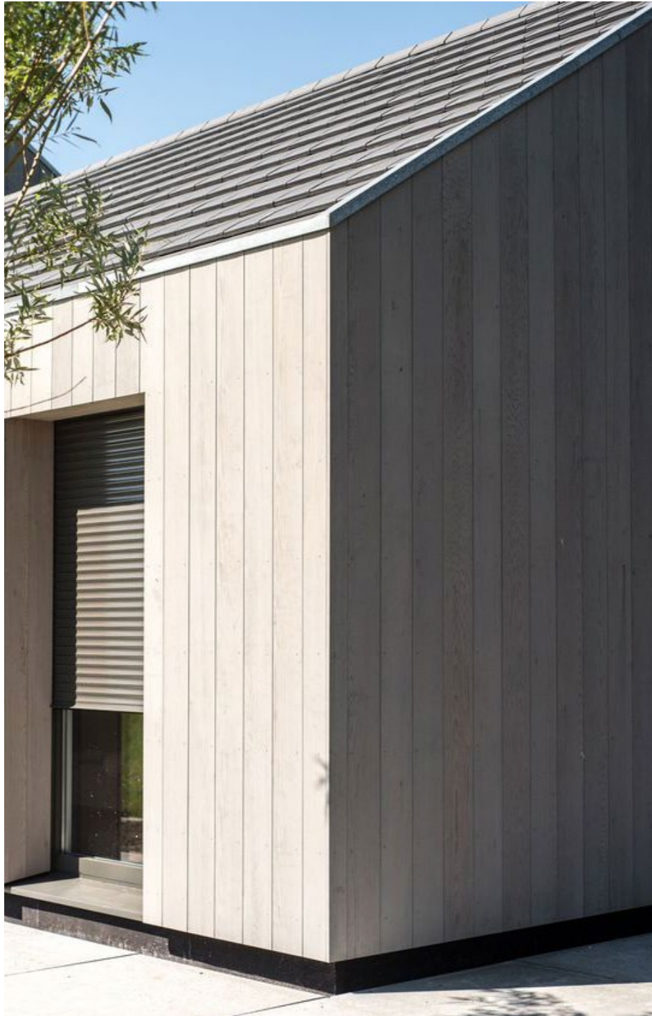
Simple timber detailing
