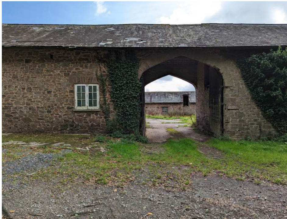
Listed barns to the South
