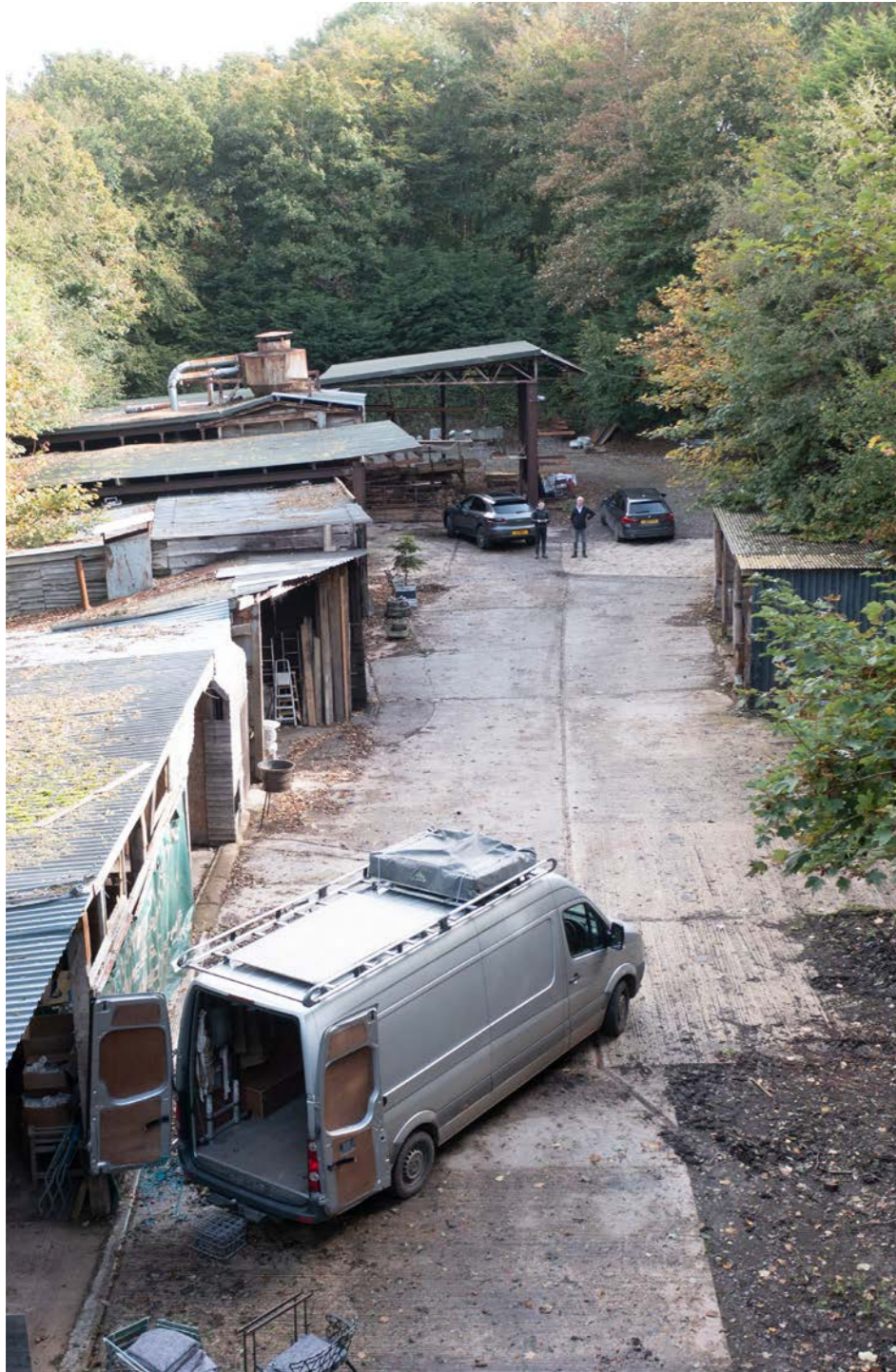
View of the storage buildings and sheds
