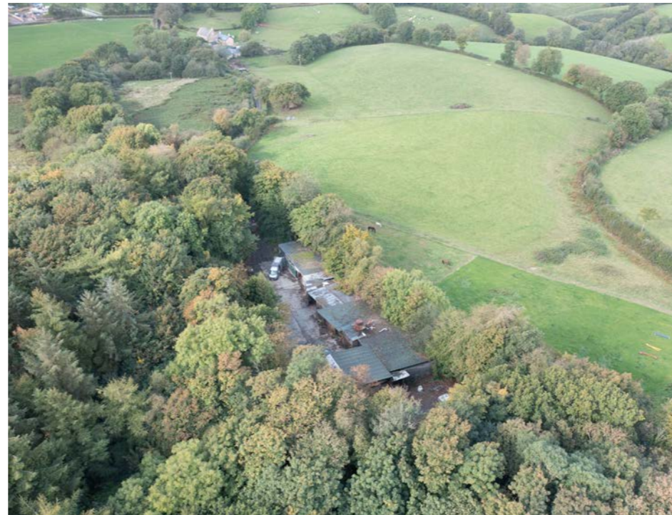
Site from the East
