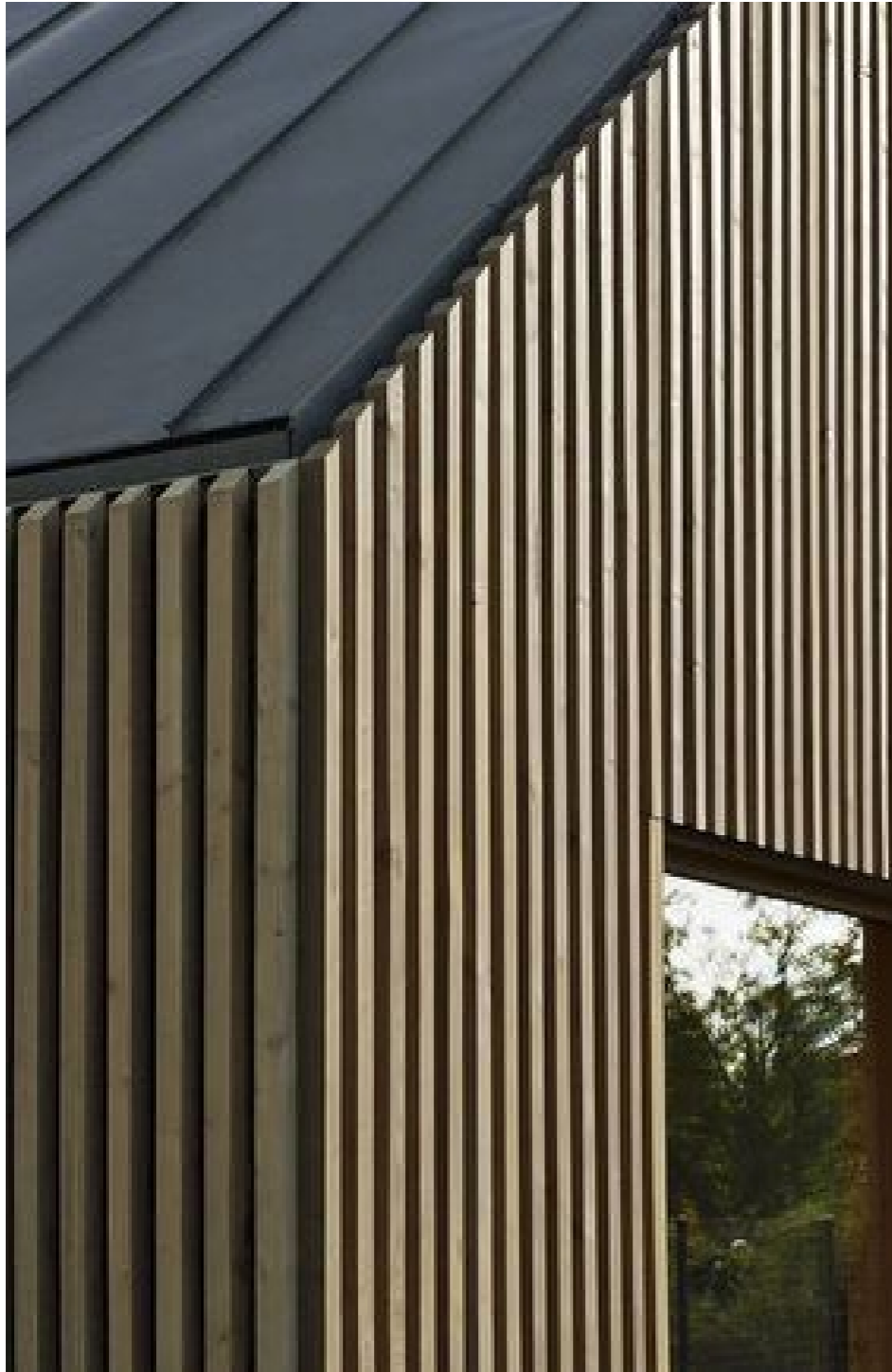
Narrow timber cladding with shadow gaps and crisp zinc roof
