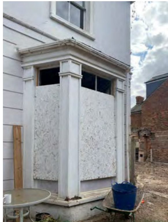
[1] Existing timber framed bay window
