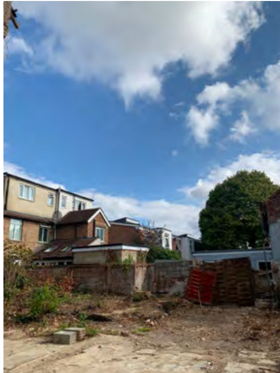
[1] View to rear garden, historically a 2 story extension was situated here. The extension had fallen into a dangerous state of disrepair and subsequently had to be removed for the safety of the site. The concrete slab of the extension is still visible. The block work wall is a section of land owned by 41 Lake Street that is intended to be given to no.3 Stewart street.
