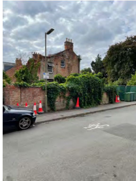
[2] View from lake Street - overgrown vegetation covers an existing pedestrian entrance - mismatch of different bricks, concrete breeze blocks and stone have been used as patchwork repairs over the years.
