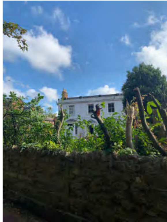
[1] View of dwelling from public footpath - level difference between the street and the front garden means that anyone in the garden is very exposed to the path. Important to note, only the ridge of the pitched slate roof is visible from the foot path due to the height of the existing parapet
