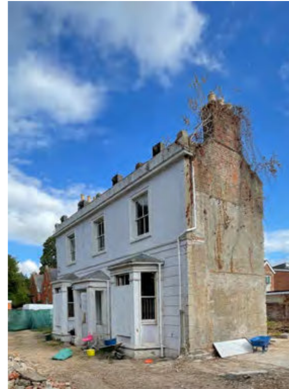
[3] South Facade shows original brick work.
