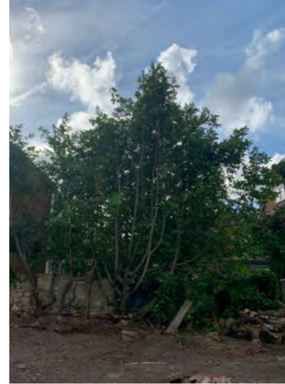
[3] View of parasitic tree from the 41 Lake street side of the boundary wall. Roots are set into the foundation of the wall.
