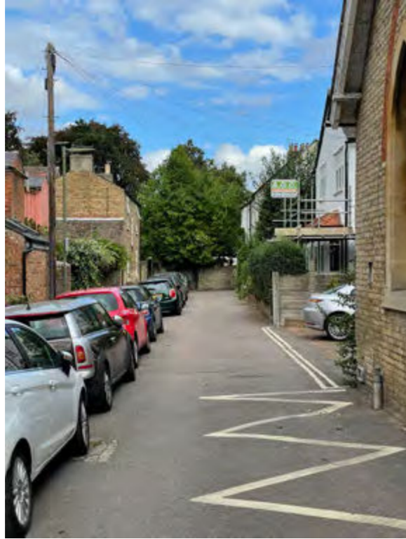
[1] View from the top of Vicarage road looking towards 41 Lake Street - street scene completely blocked by parasitic tree that has grown into the existing stone wall and significantly blocks light coming into the site.
