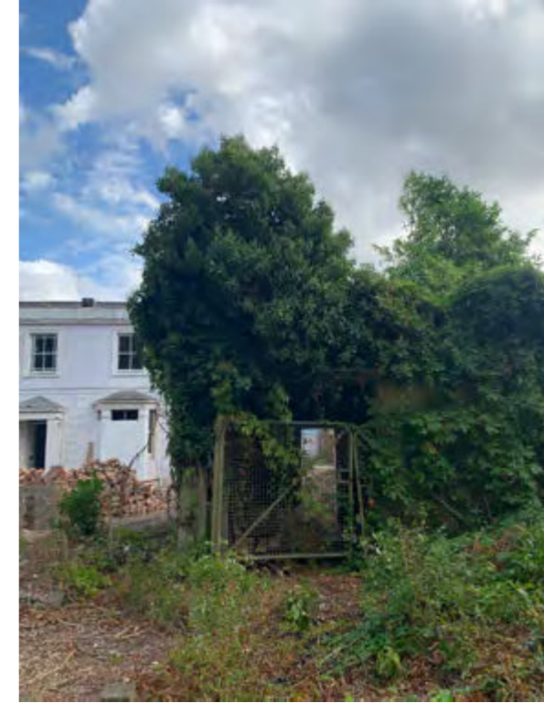
[4] View from public footpath of overgrown derelict outbuilding
