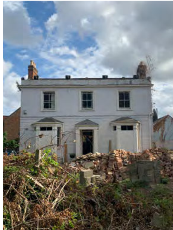
[2] View of principal facade from front garden. Both bay windows are poor quality and have been tampered with and adjusted over the years. Vegetation has started to grown in the space behind the parapet. Note: the slate pitched roof is not visible due to the height of the parapet.
