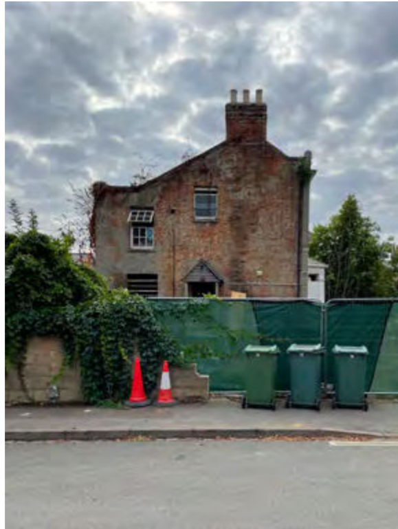
[1] View of flank elevation from Lake Street. The section of boundary wall here is concrete blockwork which has collapsed. This boundary wall is a patchwork of red brick, concrete blockwork and stone. The existing flank facade features an unbalanced window arrangement with the addition of an unoriginal side access with unsympathetic ramp and poorly constructed porch roof.
