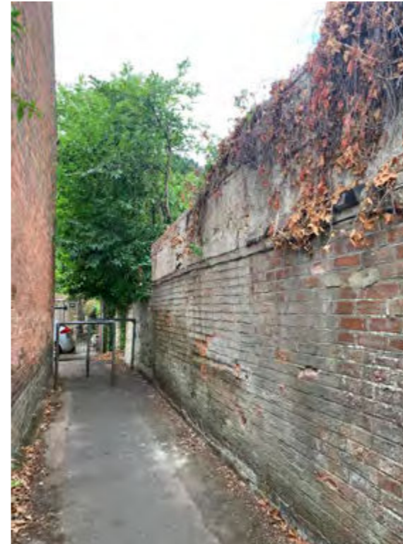
[3] View of Stewart street towards Vicarage Road- patch work of ad hoc brick additions and junction between brick and stone
